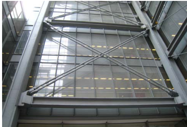
Figure 9: Exposed exterior X-braced rods
