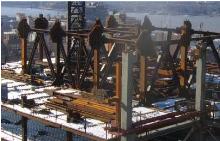
Figure 8: Core bracing during construction, courtesy of Thornton Tomasetti
