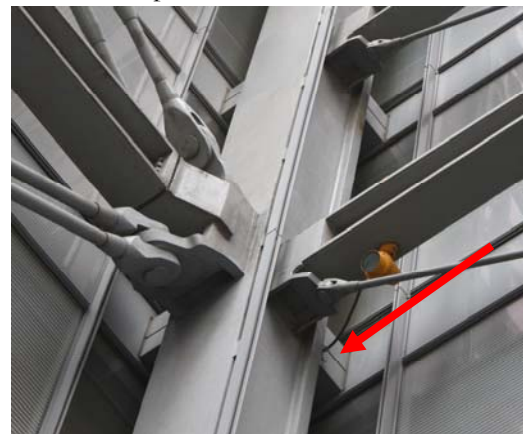
Figure 3: 'Dog-leg' penetrating building envelope
