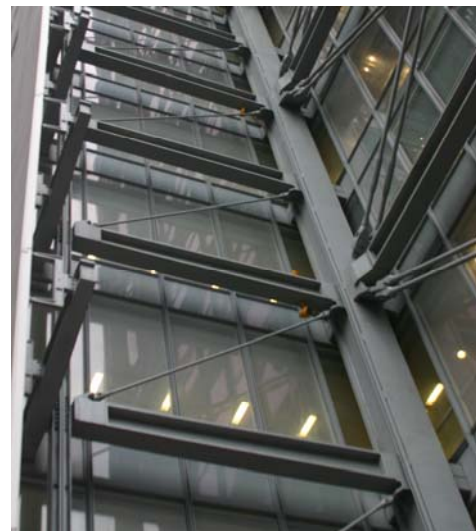
Figure 5: Cantilevered bays from exterior
